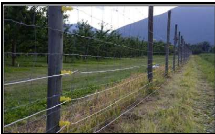
Figure 19. Ensure that vegetation below electric fence is removed or kept below wires. This is a 5 strand electric fence modified to fit with an existing paige-wire fence. Photo courtesy of Gillian Sanders
