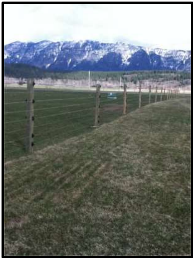
Figure 16/ A five-strand permanent electric fence set-up, using a total of eight strands of wire .Photo courtesy of Gillian Sanders
