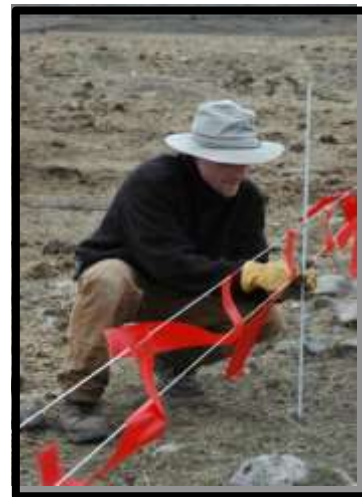
Figure 24. Setting up electrified fladry takes approximately 31.8 person hours per km. Photo courtesy of Nathan Lance
